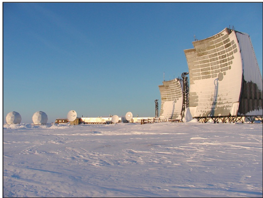
This NWS site at Hall Beach on Baffin Island, Nunavut, has two huge tropospheric dishes and several radar domes.
